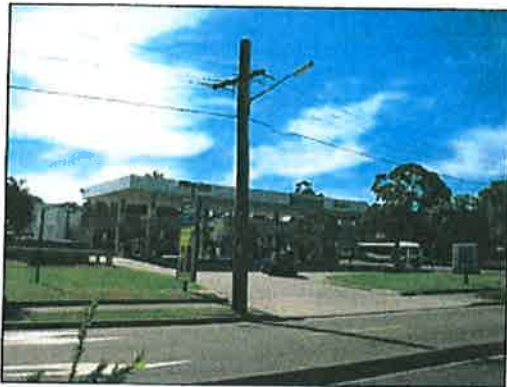
Photograph 1: View of Mobile Service Station at corner of Parramatta Road and Shaftsbury Road.
